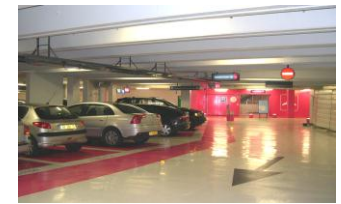
Renovation of P0 car park
